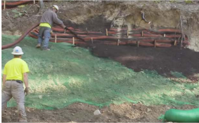
Stabilizing storm-damaged roadside banks with compost socks and blankets. (Jamaica, Vermont)
